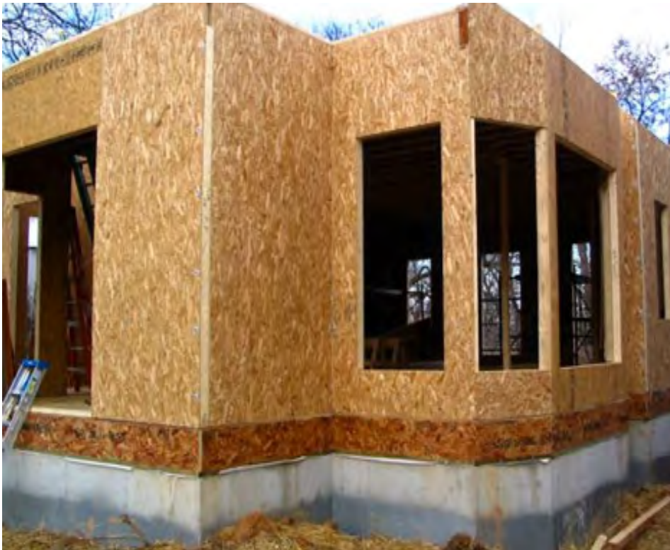
House built of OSB panels
