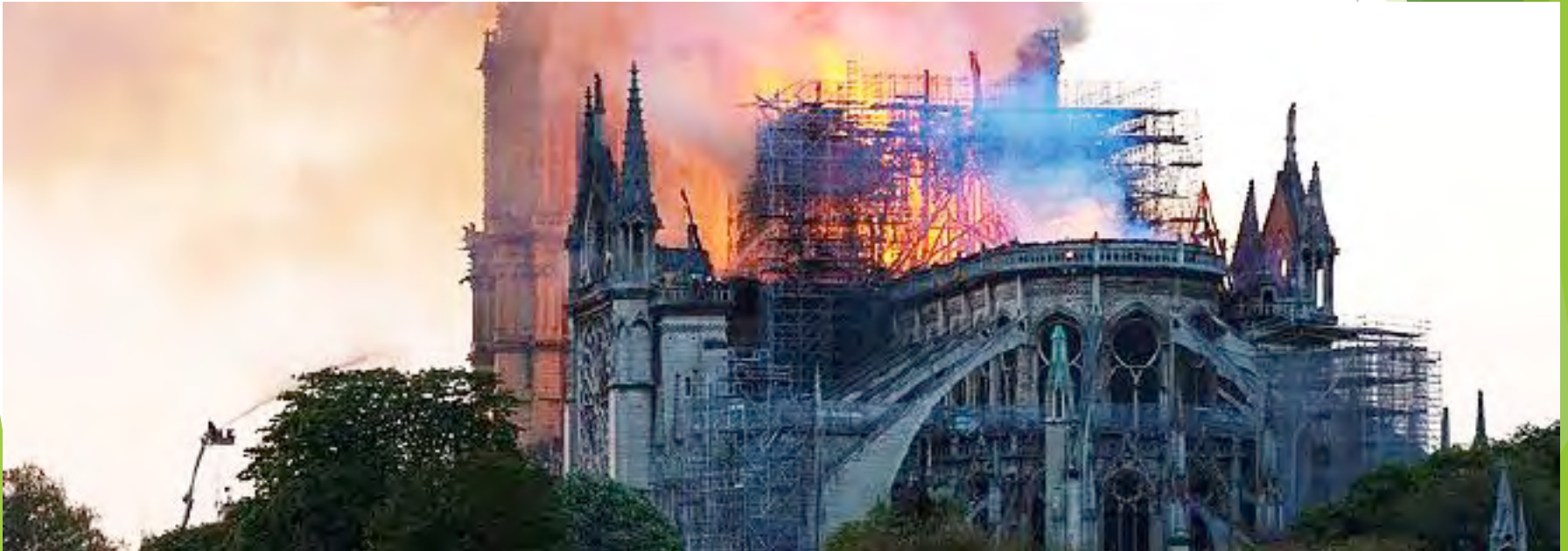
The fire broke the roof of Notre-Dame de Paris cathedral in Paris
